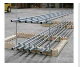
The spacing between conduits across the channel needs to be the same so that they meet up with each other when the individual runs are installed. It is recommended that installers use custom wooden jigs with notches at the spacing for each piece. They can be easily made on the jobsite with pieces of wood and customized for individual situations.
