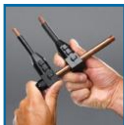
4. Slide connector/insulator assemblies onto rod.
