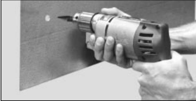
1. Drill 1/2" pilot hole using a Greenlee Kwik-Stepper® step bit.
