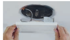
Friction clips for recessed housings
