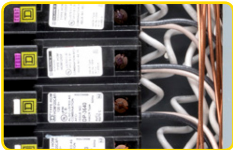
▲ Pigtail Neutral connection
