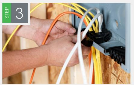
Snap on the Qwik-Grip shield when all circuits are installed
