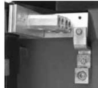
Service Grounding Lug, Bonding Strap, and Bonded Main Neutral Bus as installed on Main Devices at Job Site as Required for use as Service Equipment
