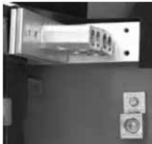
Grounding Lug and Isolated Main Neutral Bus as Installed at Factory on Main Devices
