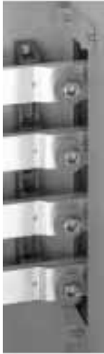
Right End of 3Ø Horizontal Cross Bus, Shown with Visi-Tite Nuts
