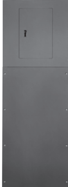
Panel skirt completely installed.
