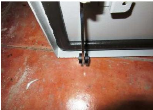
Photo 28: Spreader bar CRNG (severity B)
