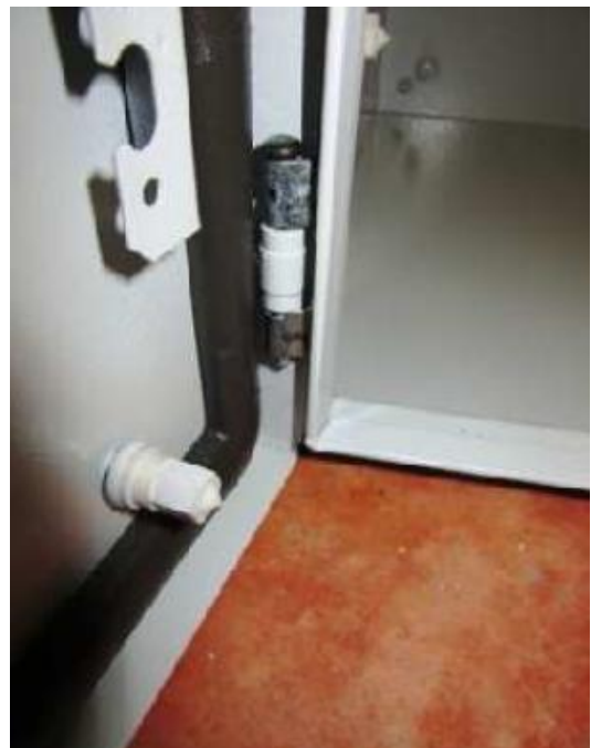
Photo 27: Hinge CRNG (severity B)
