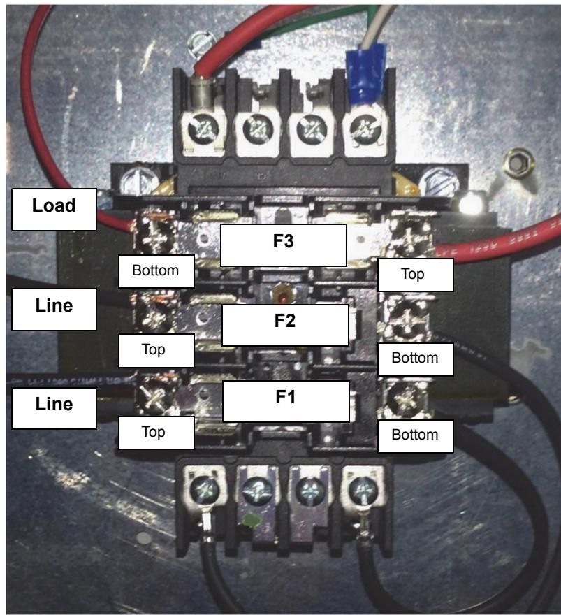
3. To confirm line isolation, repeat the test above at the top of F1, F2, and F3. There should be no voltage (0 V).
