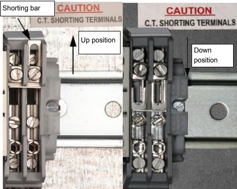
**NOTE:** The CT shorting bar must be in the DOWN position for the Automatic capacitor bank to operate.
