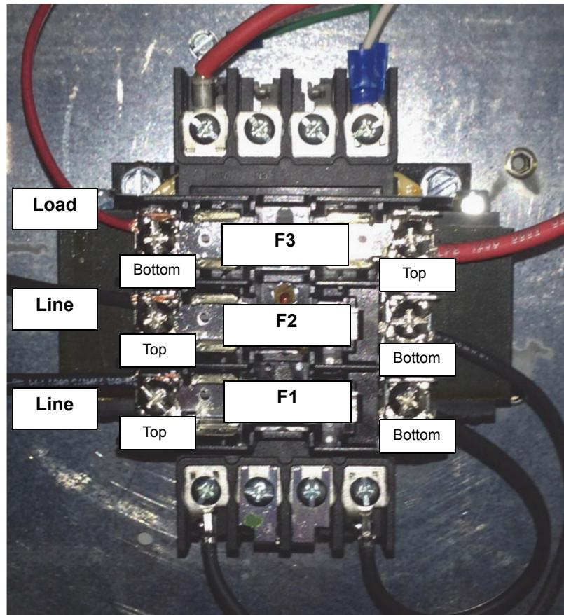
3. Repeat the test above at the top of F1, F2, and F3. There should be no voltage (0 V).
