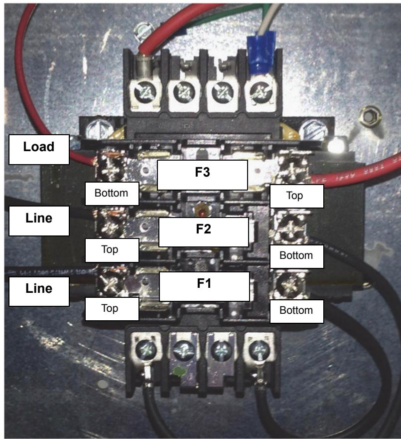
3. Test for line voltage, L-L, L-Ground at the bottom of F1, F2, and F3 control fuses. There should be no voltage (0 V).
