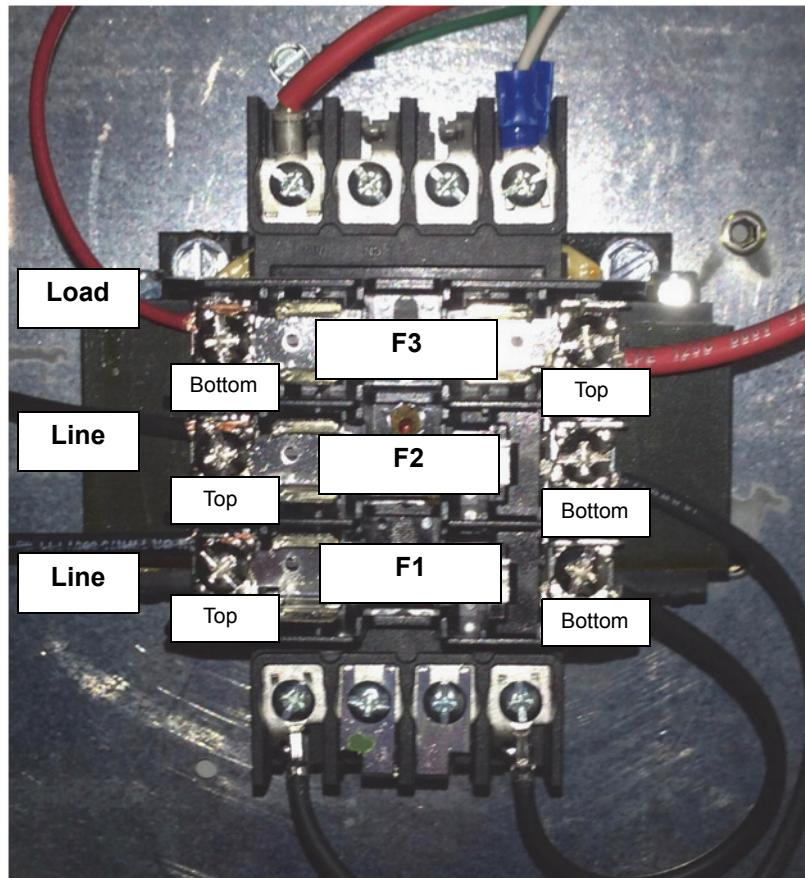
3. Repeat the test above at the top of F1, F2, F3. There should be no voltage (0 V).
