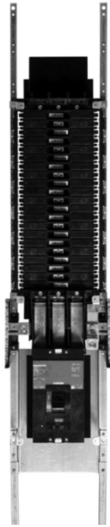
400 A LAL Main Circuit Breaker Interior
