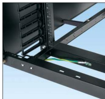
**Bond cabinets to the MCBN with single connection, reducing installation time**
