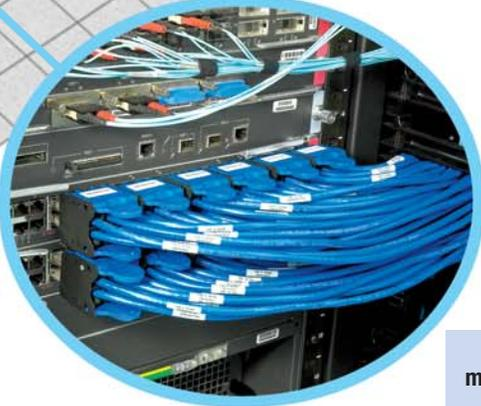
**QuickNet™ Plug Pack termination option minimizes network downtime during switch installation and maintenance**
