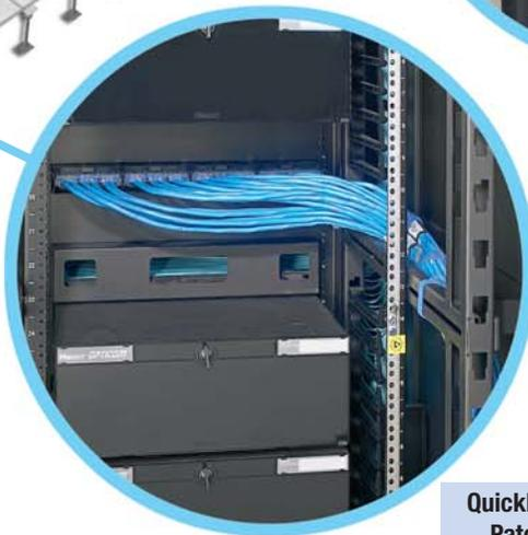
**QuickNet™ Cassettes snap in and out of QuickNet™ Patch Panels allowing easy access for moves, adds, and changes in switch or server applications**
