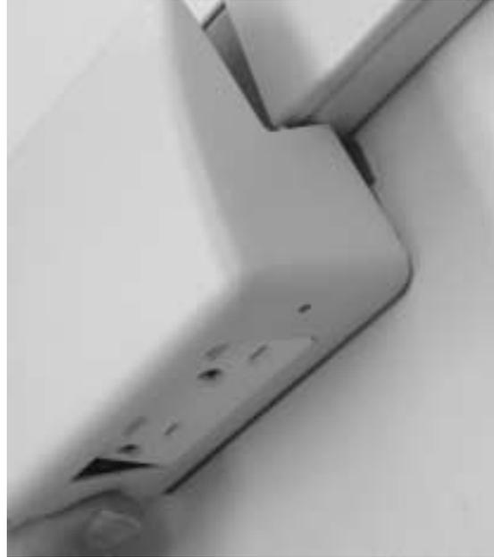
7. Secure device bracket cover with screws supplied with bracket.
