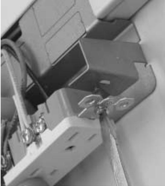
6. Snap device bracket cover onto raceway. Hook under device first, then snap the top onto the raceway.
