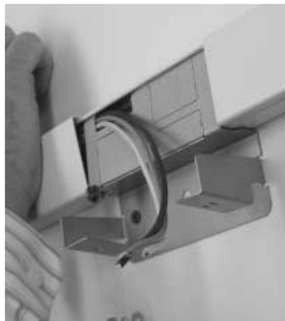
5. Wire device and mount on bracket.
