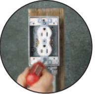
**2** Slide on a cover; no fumbling with a gasket because it's factory installed!
