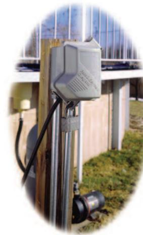
They install in less than a minute. They shrug off the worst weather. They meet new requirements for receptacles in outdoor wet locations per 2008 NEC Section 406.8(B)(1). And a few basic models cover dozens of applications, simplifying your
