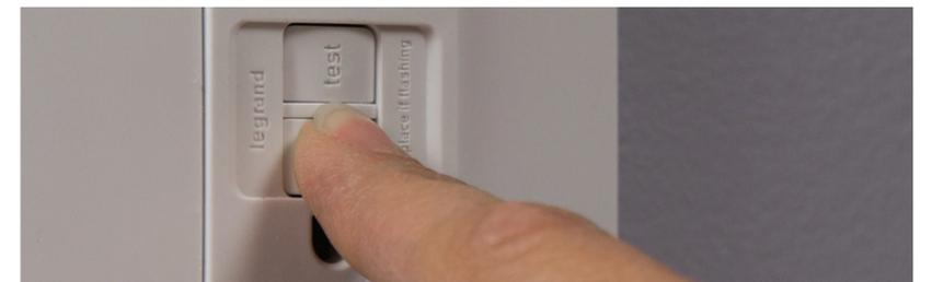
**PREVENT IT:** Without a GFCI device that is accessible and easy to see, trips can easily go unnoticed, leading to much bigger problems. Power loss to sump pumps, freezers or other important appliances can result in flooded basements or even more expensive property damage.
