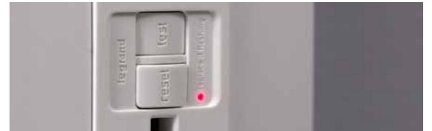
**RESET IT:** GFCI receptacles have a trip indicator light and test/reset easily with the push of a button. Breakers, however, can be confusing and unfamiliar to homeowners, making it difficult to determine the reason for the loss of power.
