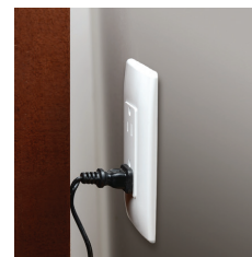
Furniture pushed against the plug of an appliance cord can stress conductors and damage insulation.
