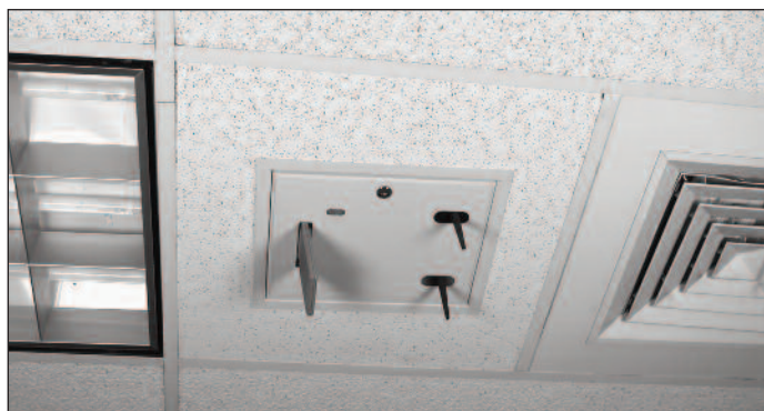
WAPE Wireless Access Point Enclosure installed in a drop ceiling.
