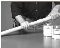
Usually the solvent-cemented joint will be strong enough to install immediately, but in low temperatures and high humidity, extra time may be required before moving the pipe to install it permanently. Solvent cemented joints appear to “set up” instantly, but will take 24 hours to cure properly. After this time, the solvent-cemented joint has completely cured and is waterproof. Kraloy cement is available in half-pint, pint, quarts and one-gallon containers.
