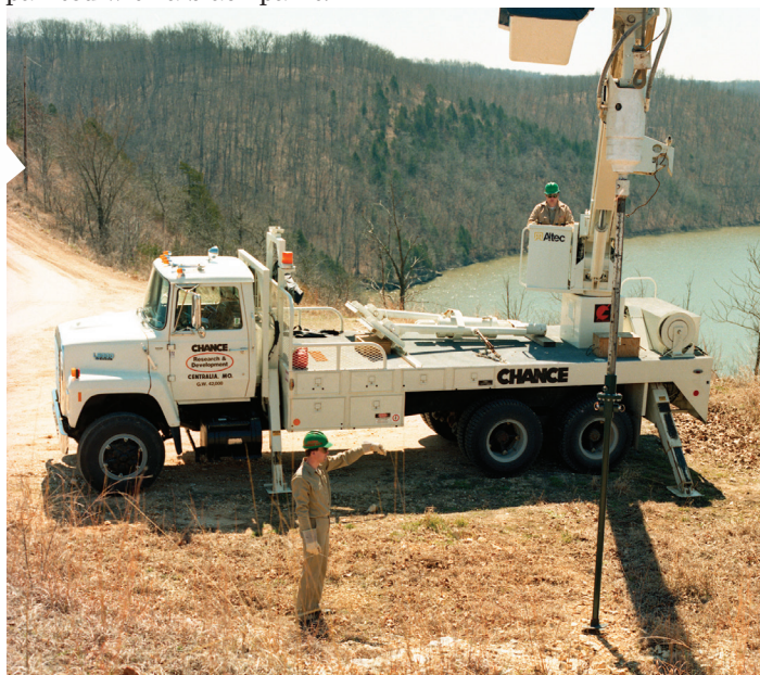
PISA ® anchor installation takes about 5 minutes with two workers.
