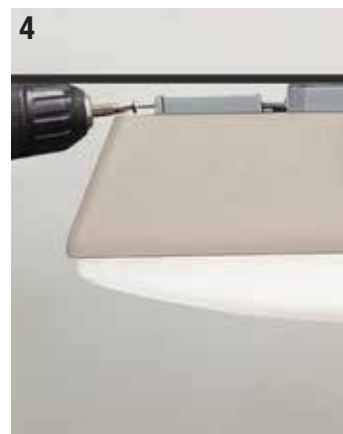
Two mounting screws close and secure fixture to the mounting bracket.
