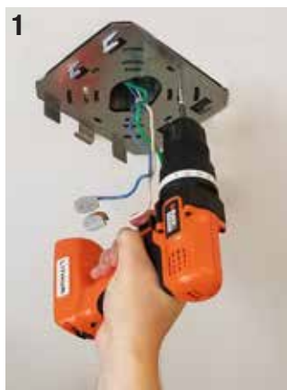
Mount plate to junction box.
