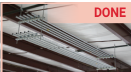
Level, tighten lock nut
