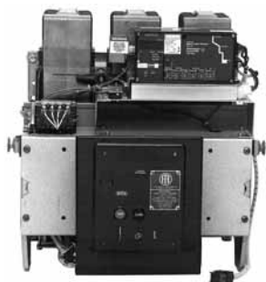
K-1600 Breaker Retrofitted with Digitrip RMS 810 Retrofit Kit
