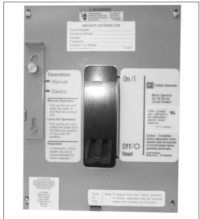
Figure 3-3 Motor Operator in Manual Position
