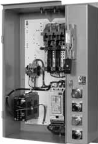
Type 3R Fused S801+ /T/ Soft Starter
