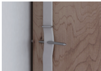
Inadvertent nails can puncture wire behind wall
