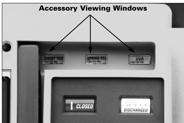
Figure 1 Through-the-Window Electrical Accessories
