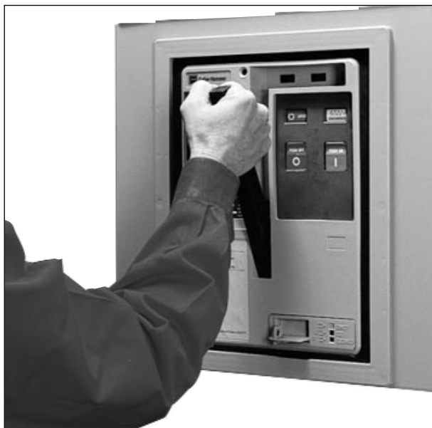
Magnum Circuit Breaker Being Manually Charged
