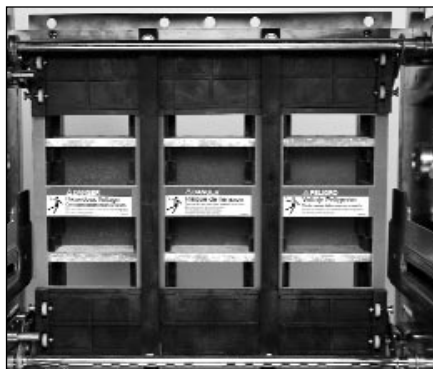
Figure 13 Safety Shutters in Open Position
