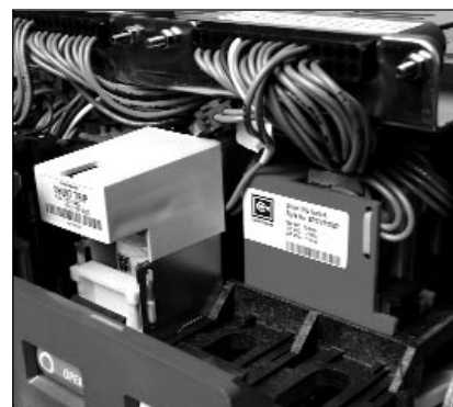
Figure 3 Shunt Trip Switch Installed
