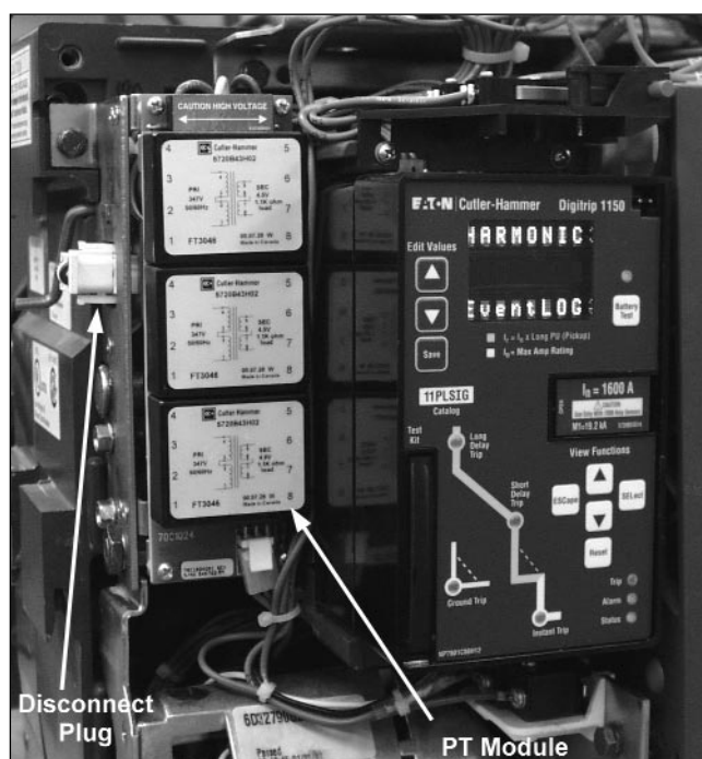
PT Module with Dielectric Disconnect Plug
