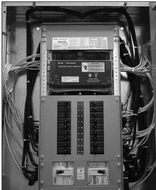
Figure 3.2.6 Stacked Pair of IQ Multipoint Energy Submeter II in a Cutler-Hammer Type PRL3a Panelboard
