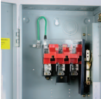
Double-Throw Switching Neutral Safety Switch (upper switch base assembly is shown)
