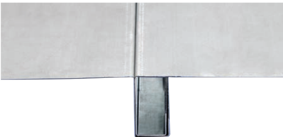
Interlocked FM planks (end view)
