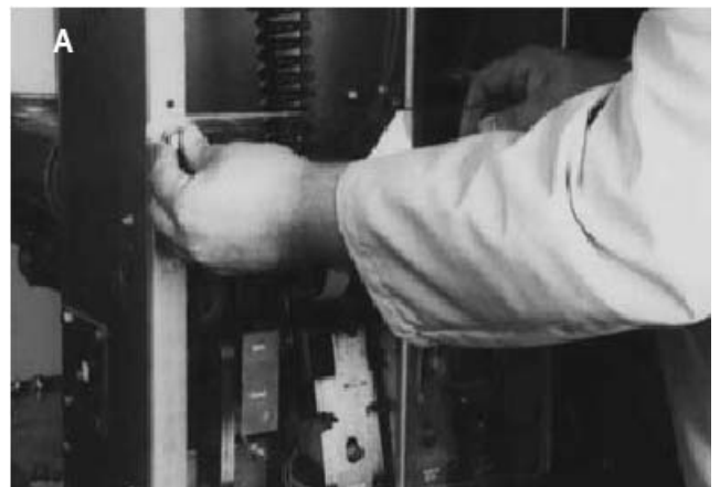
Figure 6-9 Attaching CloSure™ Test Tool at Hole “A”
