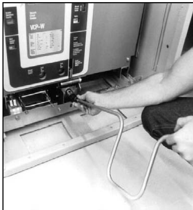
Figure 4-6 Engaging Levering-In Crank
