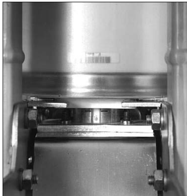
Figure 6-3 Vacuum Interrupter Showing Contact Erosion Indicator with Breaker Closed (Indicators are Checked Only When Breaker is Closed)
