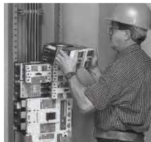
Panelboard Installation
