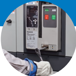
Levering Magnum DS breaker through the door
