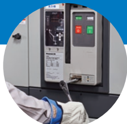
Levering Magnum DS breaker through the door
