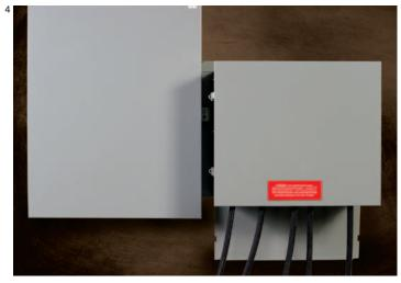
1. 100A and 200A QCDT Receptacle Compartment with Generator Plugs Connected
