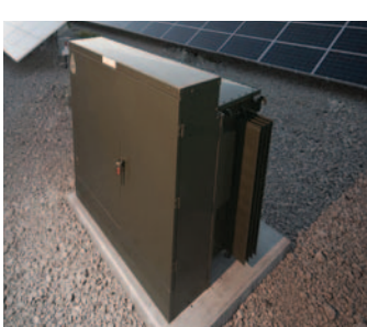
Medium voltage step-up transformer
