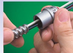
Snap fitting onto cable and twist clockwise.
