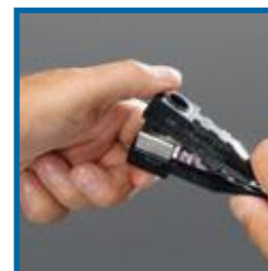
2. Snap Multi-Tap insulators over connectors.
