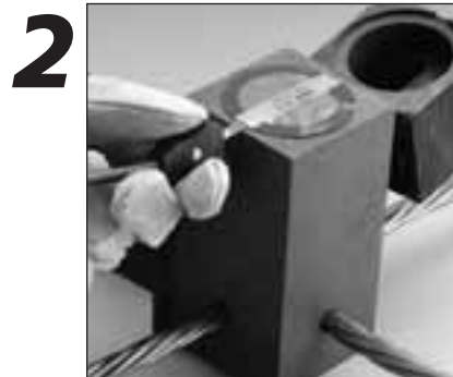
Attach control unit termination clip to ignition strip
