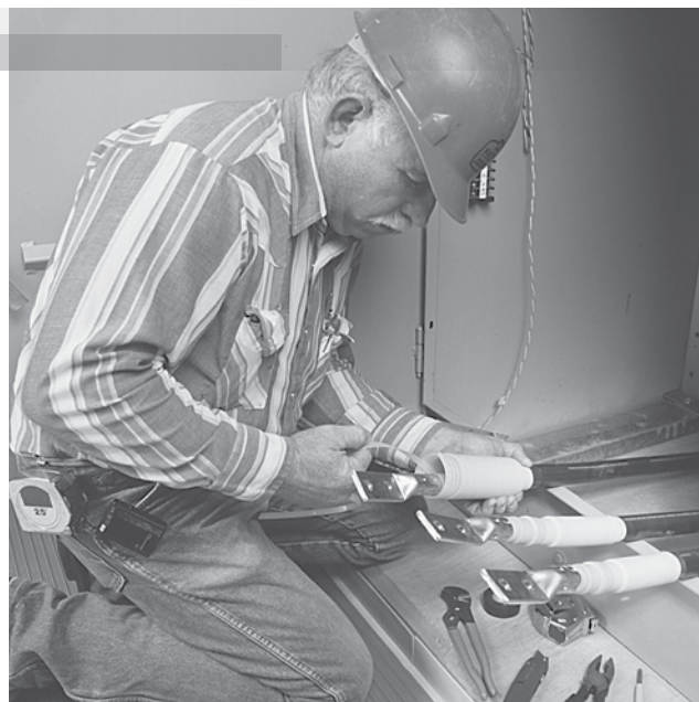
3M™ Cold Shrink QT-II Indoor Termination
